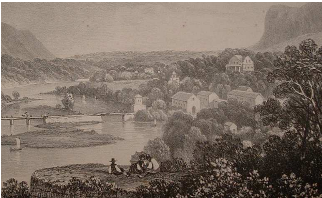
Figure 4.8 Grande Rivière Nord-Ouest T. Bradshaw (Views in the Mauritius, 1852). The convicts were housed in the buildings nearest the river.
