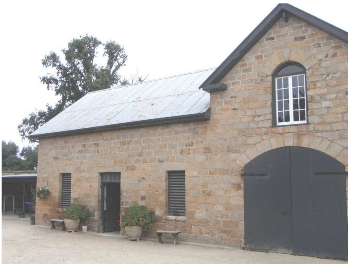
Figure 7.3 The barn at Rossiville, built in 1838 Author's photo 2011.
